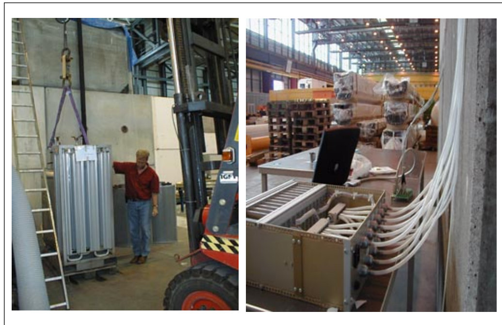
Figure 5.2 Weighting the dewar, Johan Bremer (left) and Thermocouples and Oxygen detectors (right)
