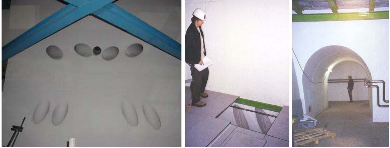
Figure 12. Left: The holes for the trigger cables on the ATLAS side of the USA15 wall. Middle: The holes for the trigger cables enters the USA15 cavern under the floor boards at ground level and the first floor. Right: The entrance of the UPX14 tunnel in USA15.
